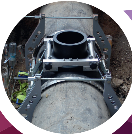
Branch Saddle installed on PE pipe with spigot outlet
