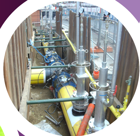
Saddle used for live by-pass during equal tee installation
