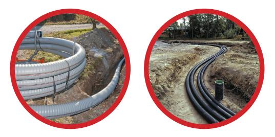
Choice of bedding and backfill materials, design of cover depth to accommodate traffic loadings and compaction requirements all follow the same principles as polymer pipes for water supply systems. Manufacturers provide detailed guidance on this aspect.
