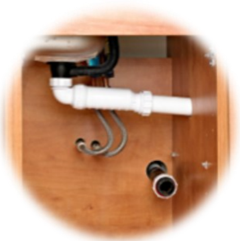
Domestic sink with waterless trap
