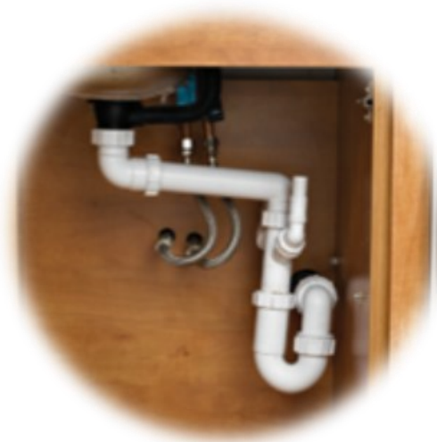
Domestic sink with water-seal trap
