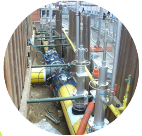
Saddle used for live by- pass during equal tee installation
