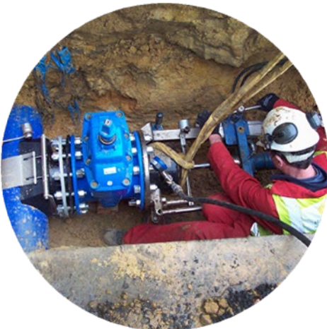
Saddle used for new connection to existing infrastructure
