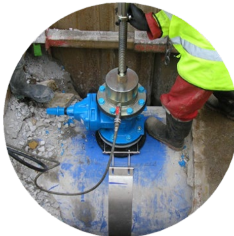
Saddle used to introduce air valve to a close fit PE liner through iron pipe
